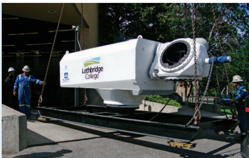
Workmen assemble the wind tower at Lethbridge College.
