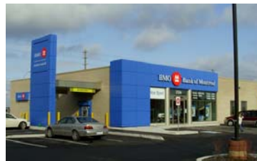
Oakville, Ontario branch, one of up to 53 branches in Ontario & Alberta to be bullfrogpowered™, using renewable energy sources like wind power and low-impact water power
